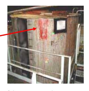
Corrosion on plates of heat exchangers indicates possible contamination
